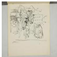
Oslo City Hall Under Construction Edvard Munch 1928-1930 Pen MM.T.00195-097
