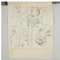
Oslo City Hall Under Construction Edvard Munch 1928-1930 Pen MM.T.00195-105
